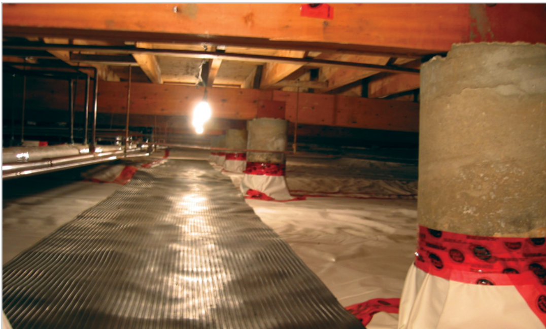
Figure 2 Crawl space after remediation
