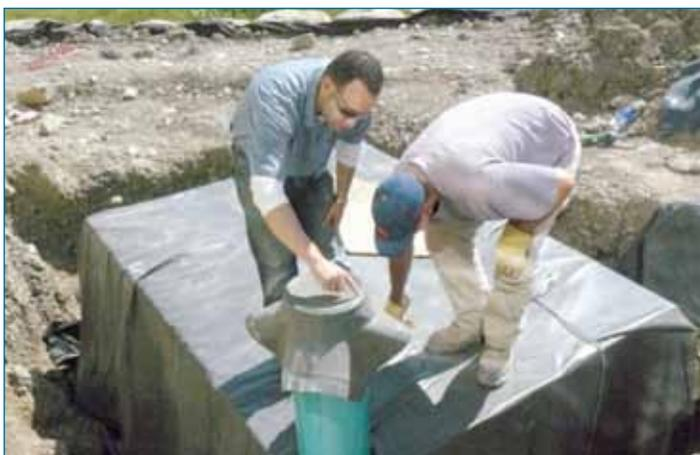
**Figure 4** Cistern in cavity, wrapped and seam-sealed
