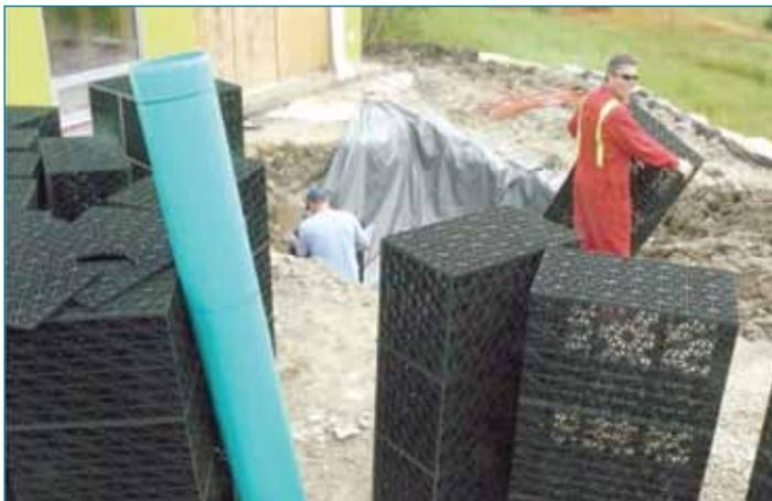
**Figure 3** Crate assembly to form cistern cavity under driveway
