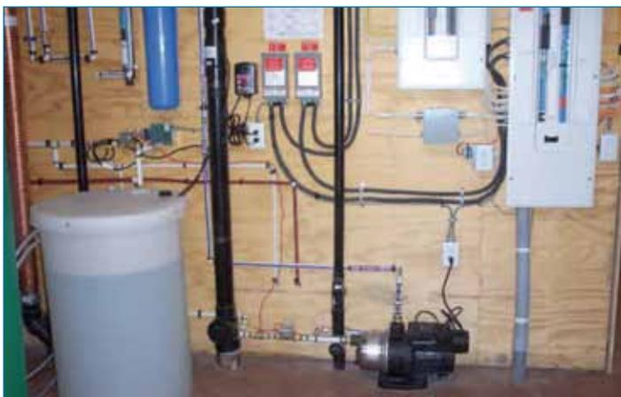
**Figure 5** Mechanical room components of rainwater collection system
