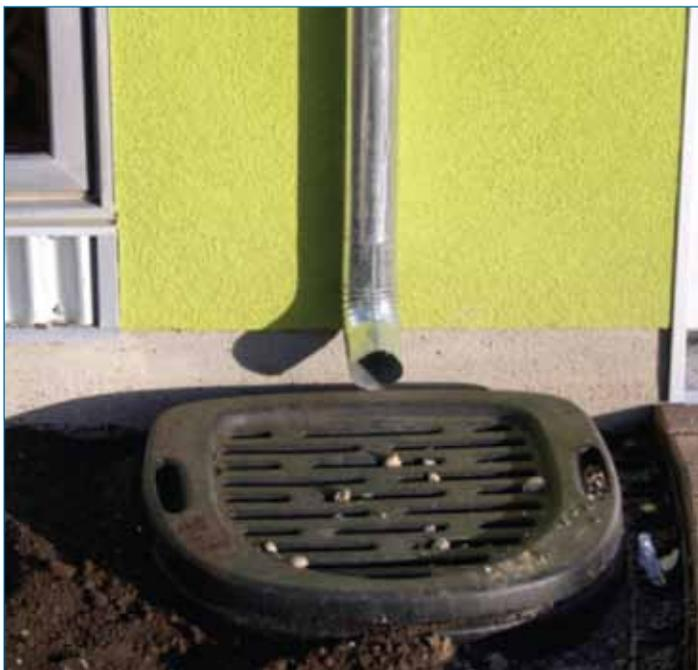
**Figure 1** Filter component at downspout
